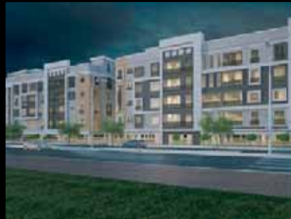
Gardenia Residence North Jeddah.
